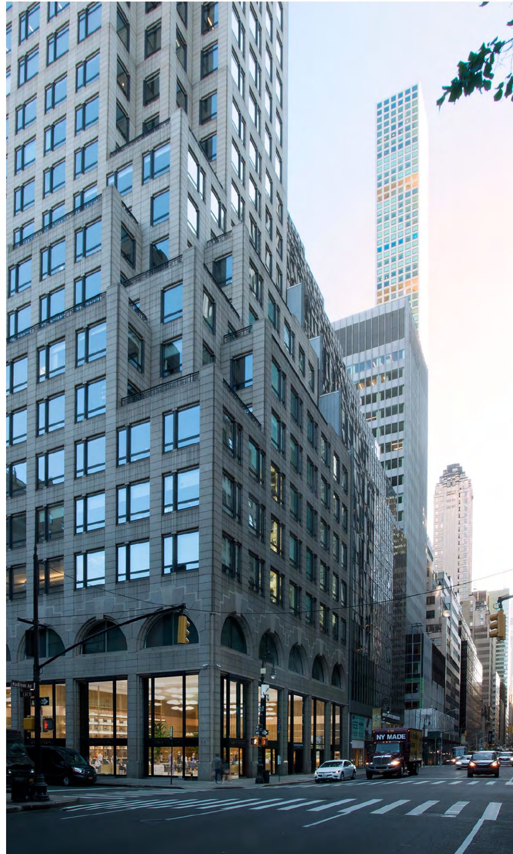
Building Northwest Corner
