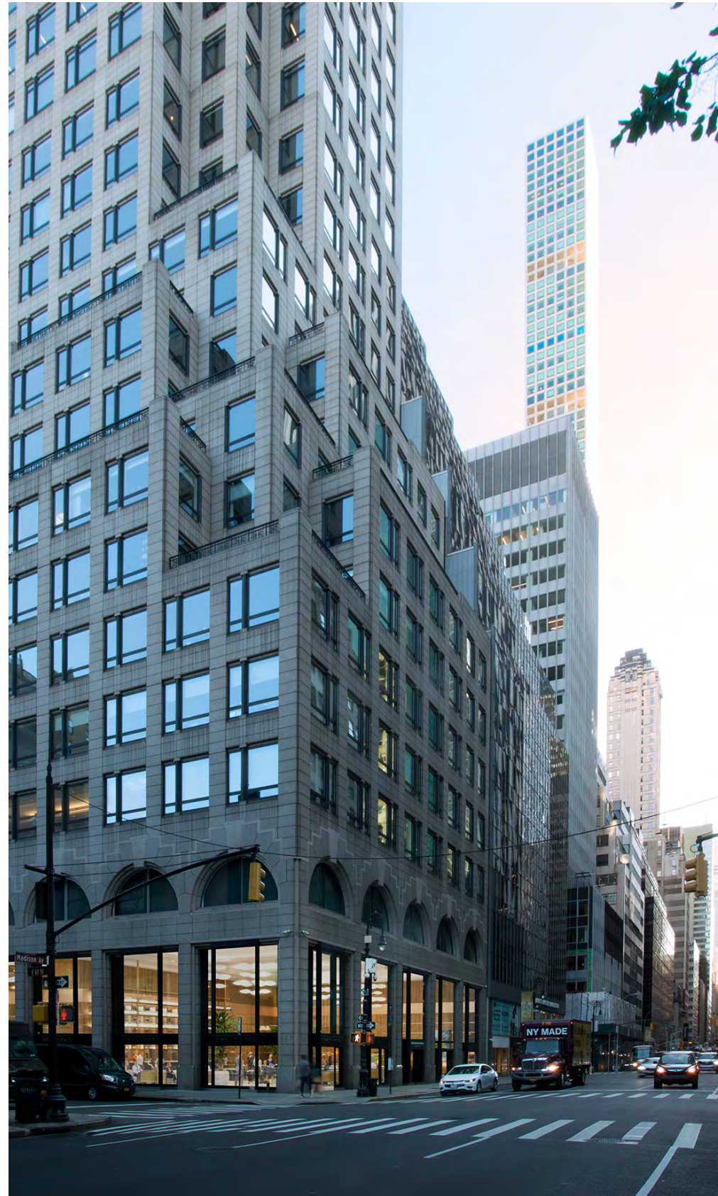
Building Northwest Corner
